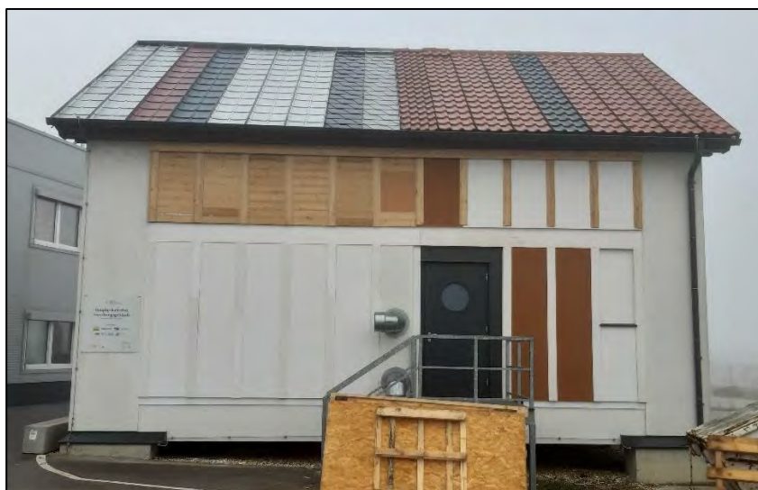
Figure 6 : Photo of the north facade.
