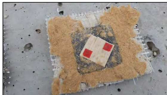
Figure 43: Removed render layer of variant N 2.3 (bright render) with Balsa sensor and wood fibre residues. No fungal mycelium visible.
