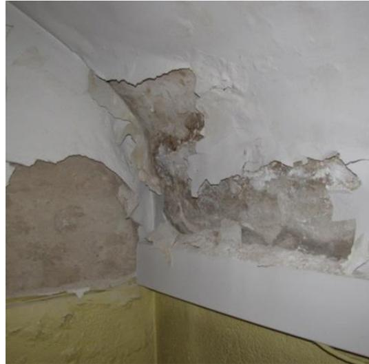
Coating and plaster are spalling off
