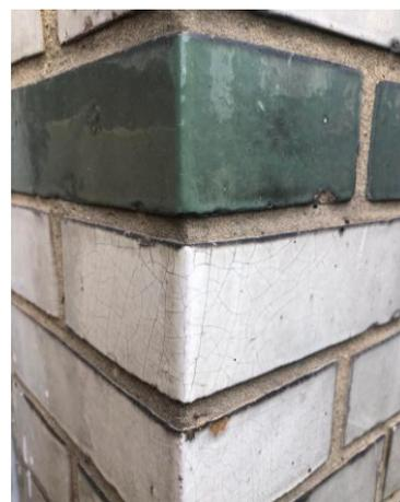
Glazed bricks (early 20th century); masonry can still dry out through the joints in between the bricks
