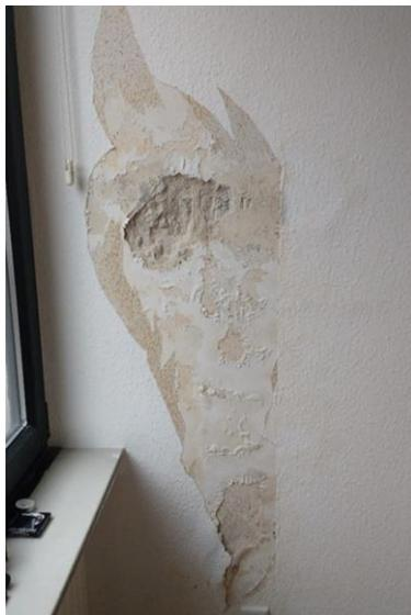
After removing wall paper visible mould stains
