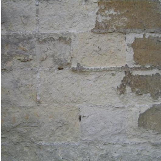
Degraded limestone due to acid rain
